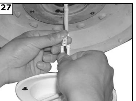
Plug white wire from fan to white wire from light kit. Then plug black from fan to black from light kit.
